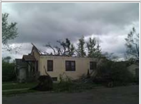
Home damage in Minneapolis, MN
